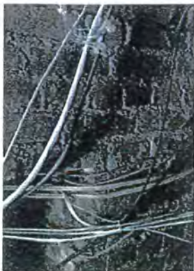
Romex and Other Cables in Crawl Space
