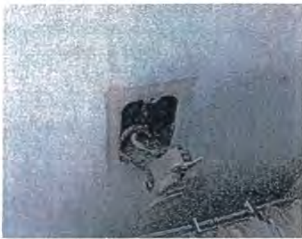
Receptacle without Ground Wire
