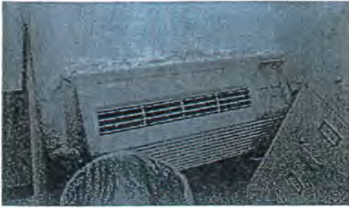
Thru-wall Mechanical unit
